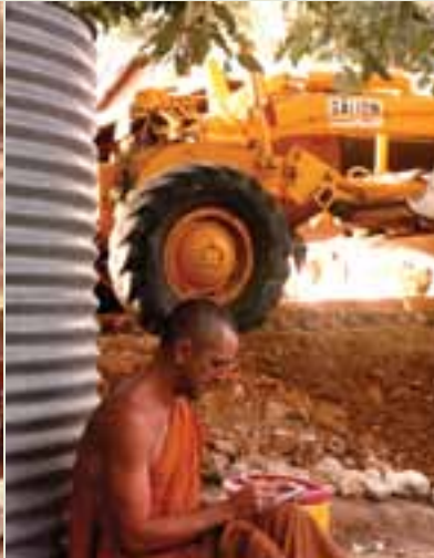
Grading the gravel by the dining hall, 1985
