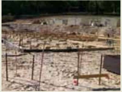
Meditation hall formwork, 2 May 2008
