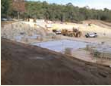
Cottage foundations, 29 Mar. 2008
