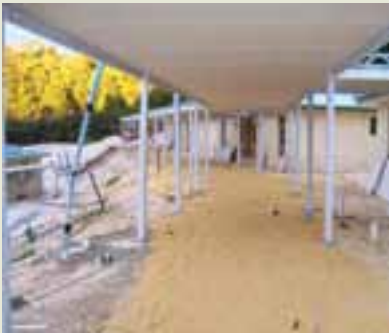
Walkway to the cottages, 29 Jan. 2009
