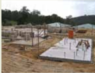
Dining complex foundations, 14 Sept. 2008
