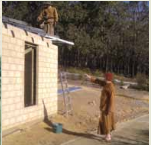
Ajahn Brahm supervising the construction of the teacher's cottage at Jhana Grove, 2011
