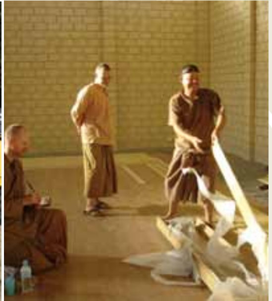
Monks working on the floor of the main hall into the early hours to complete it on time
