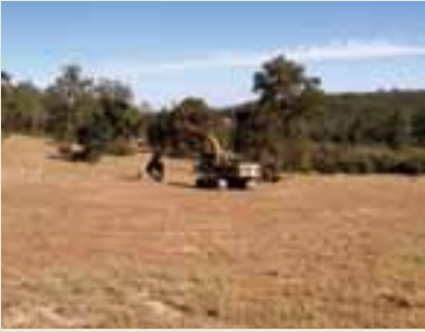
Clearing the ground, 16 Nov. 2007
